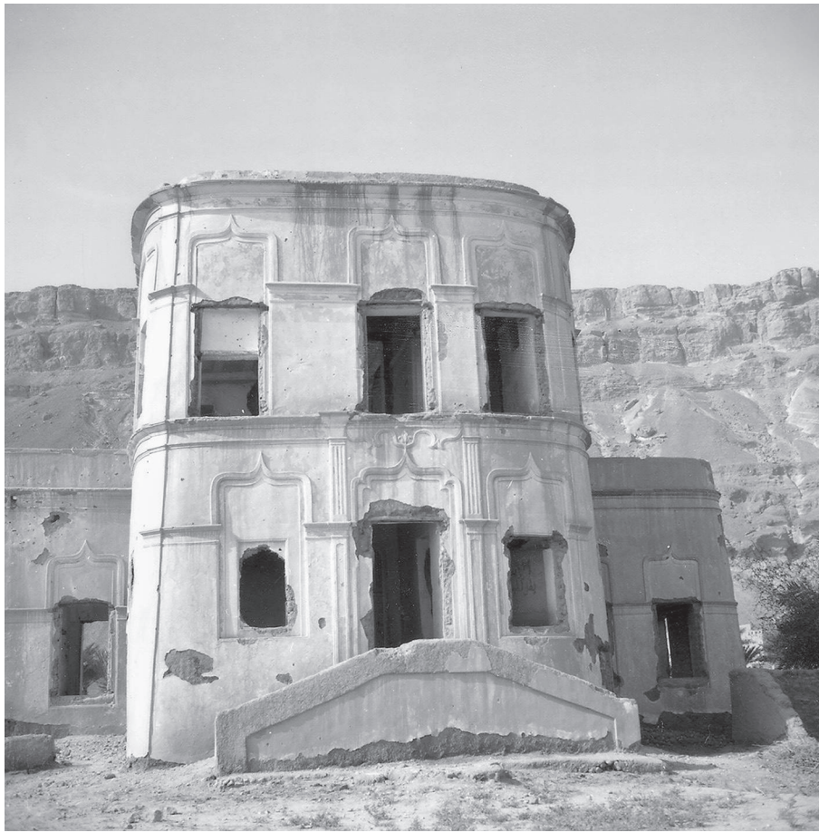
FIGURE 7.4 Custom House Built by the Kathiri. CREDITS: CHRISTIAN DARLES.
