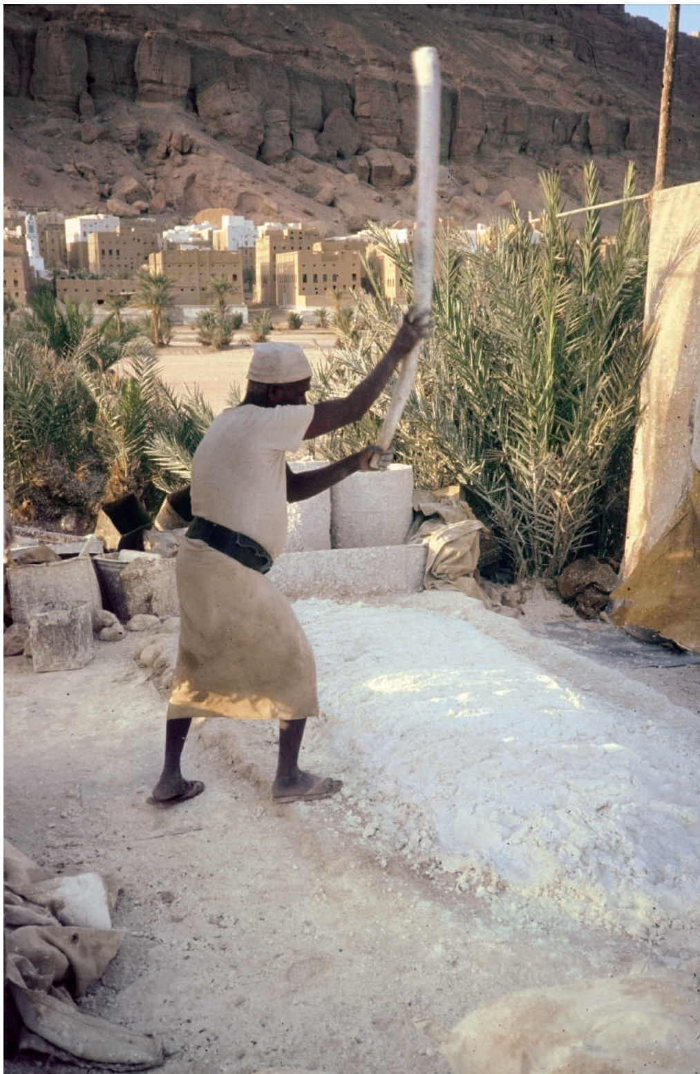
FIGURE 7.18 Lime-based Ramad for Waterproofing the upper Parts and Basements of the Houses. CREDITS: CHRISTIAN DARLES.
