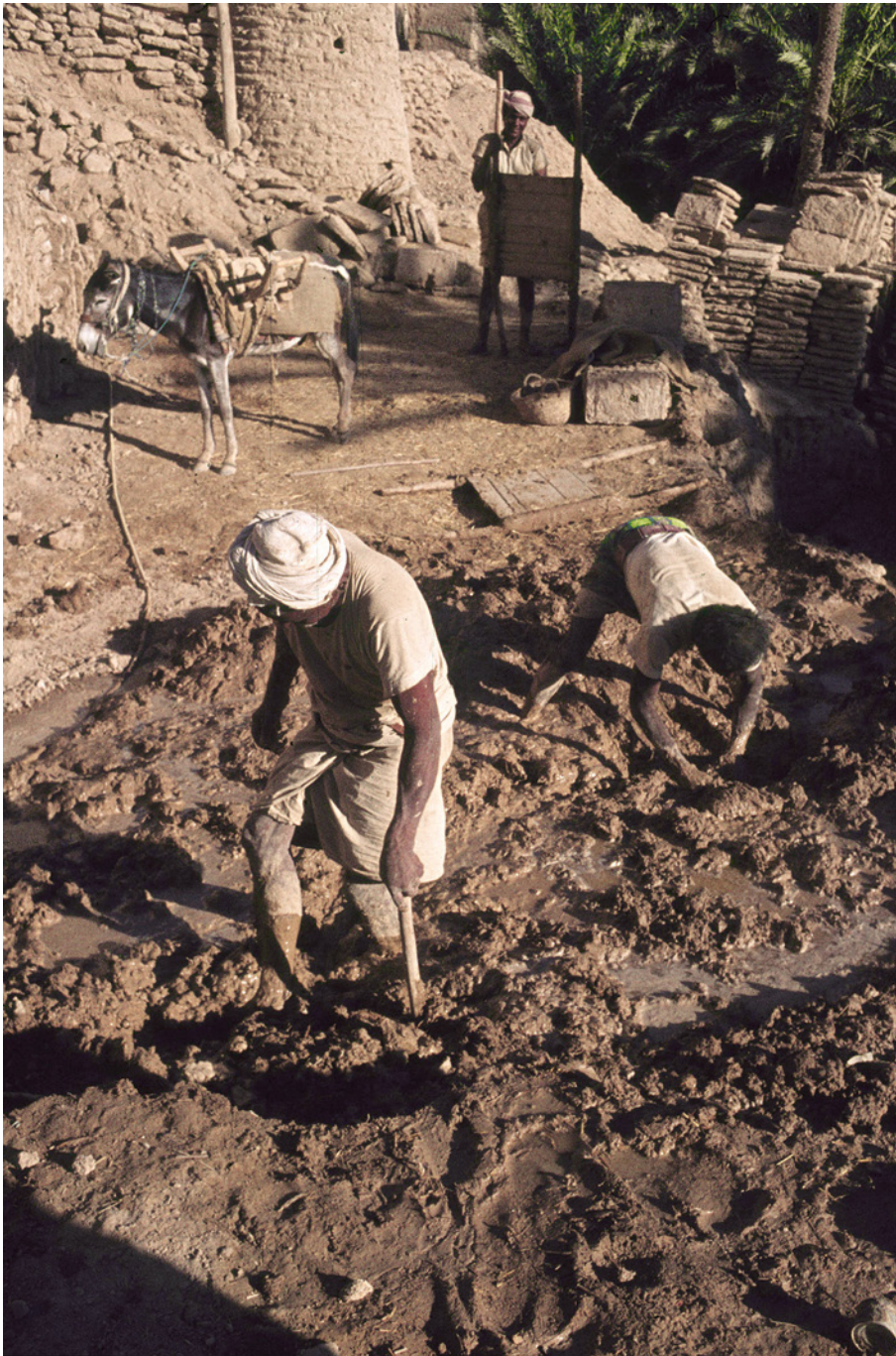
FIGURE 7.8 Worker from Shibam who is treading the earth CREDITS: CHRISTIAN DARLES.
