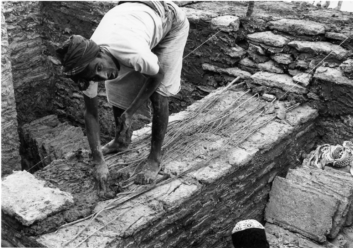
FIGURE 7.19 Branches and timbles enable the clamping of the walls CREDITS: CHRISTIAN DARLES.
